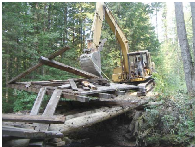
Removing Busk Bridge
