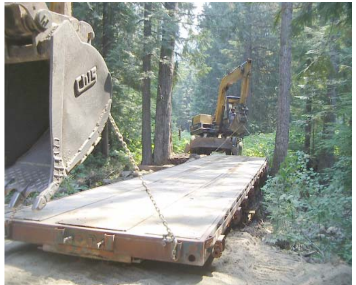
Moving the bed onto the footings
