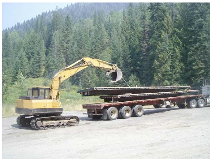
Truck beds to bridges
