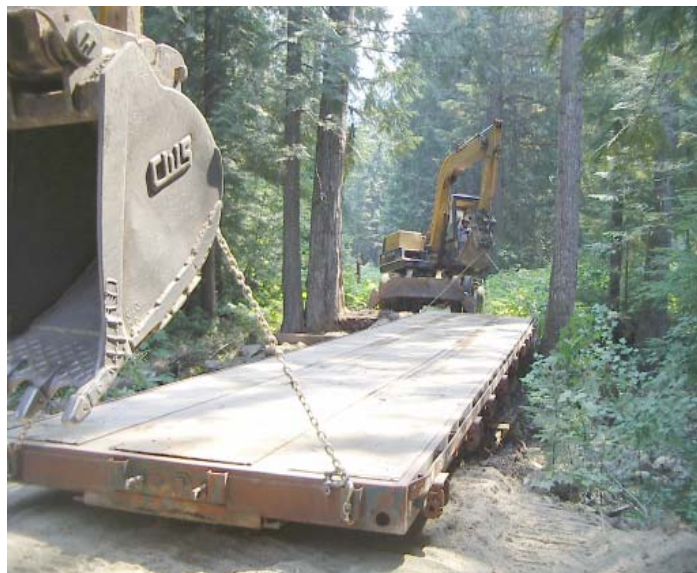
Moving the bed onto the footings
