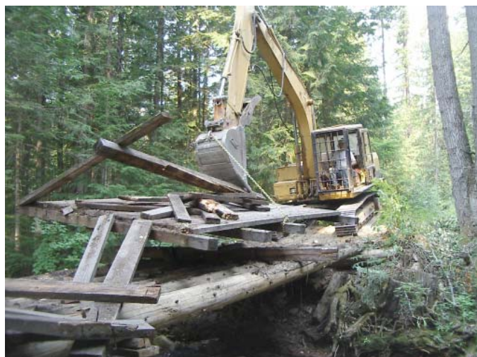
Removing Busk Bridge
